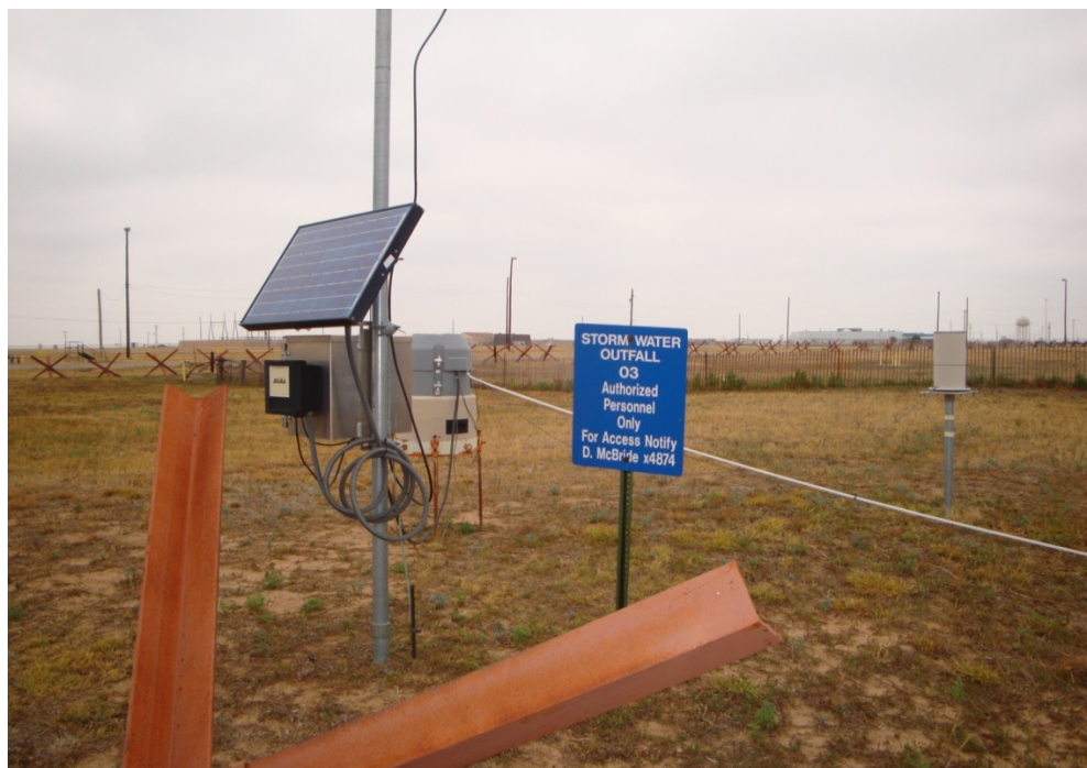
FIGURE 9.6 — Storm Water Outfall 03
