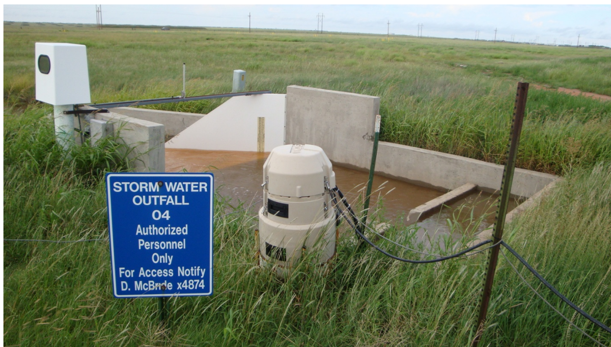
FIGURE 9.7 — Storm Water Outfall 04
