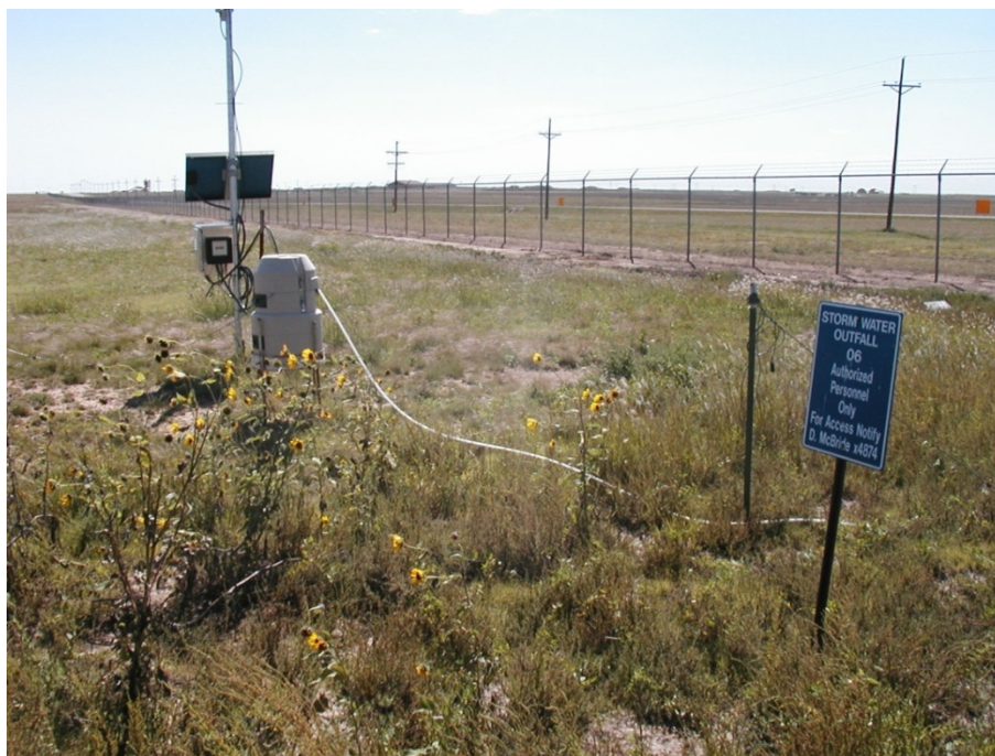
FIGURE 9.4 — Storm Water Outfall 06
