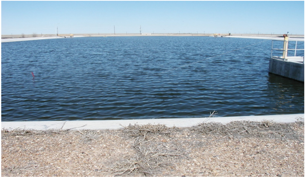
FIGURE 8.2 — Wastewater Treatment Facility, Facultative Lagoon
