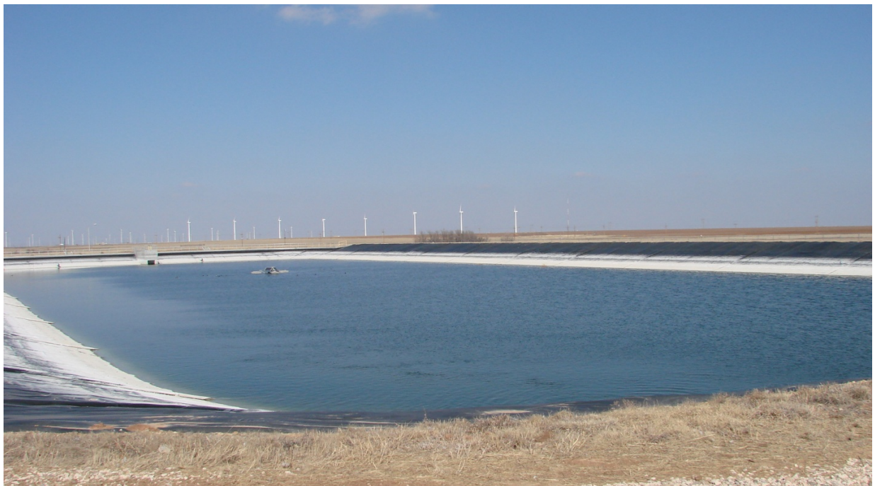
FIGURE 8.3 — East Wastewater Storage Lagoon
