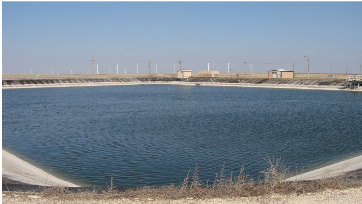
FIGURE 8.4 — Wastewater Storage Lagoon
