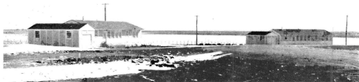
The colorful staff houses add a touch of hominess to the plant site. Shown at top is the residence of Major Irvine and below that of Capt. Ben Davis, left, and Lt. J. B. Hart, right.
