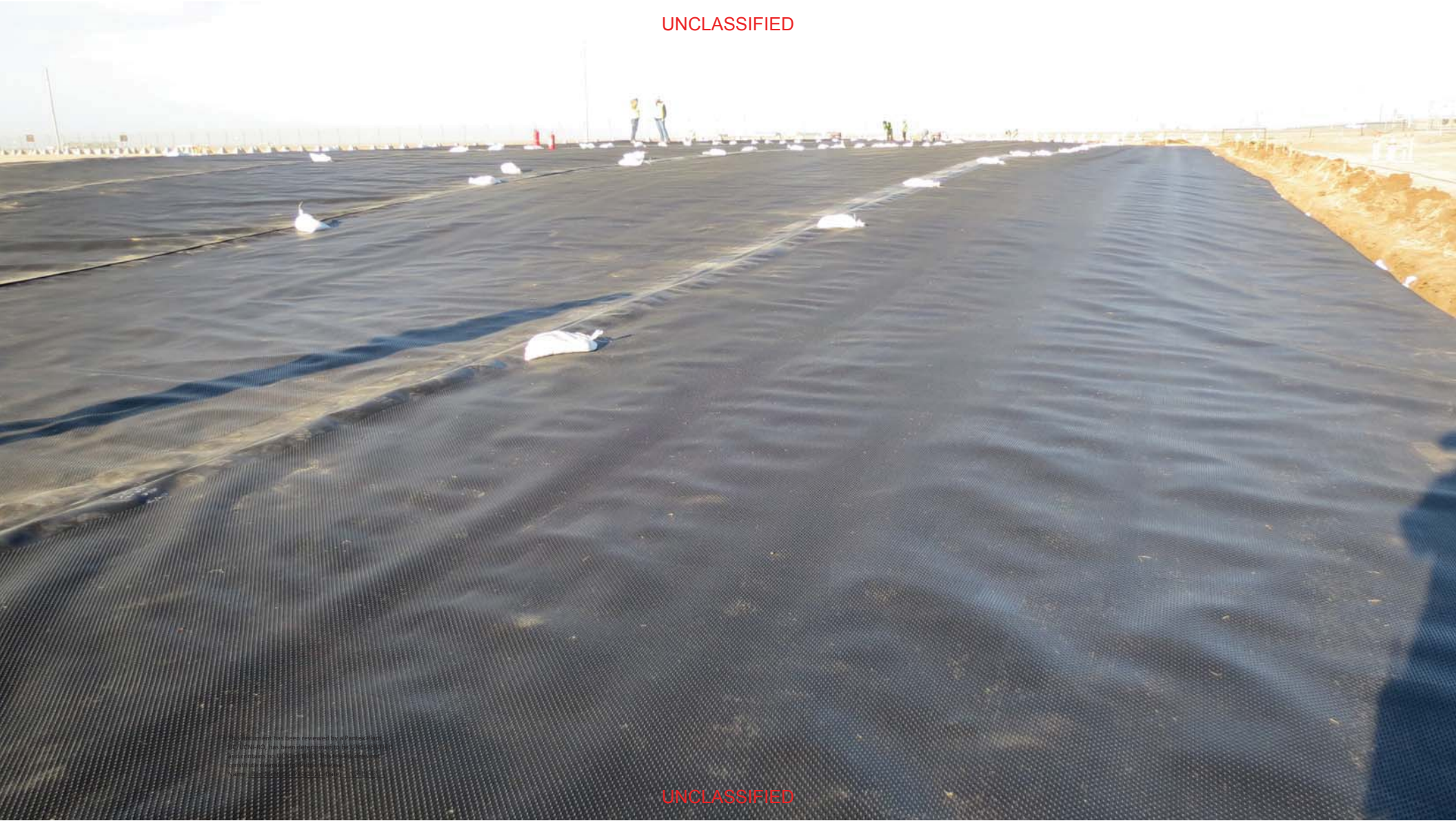
Geomembrane Installed
