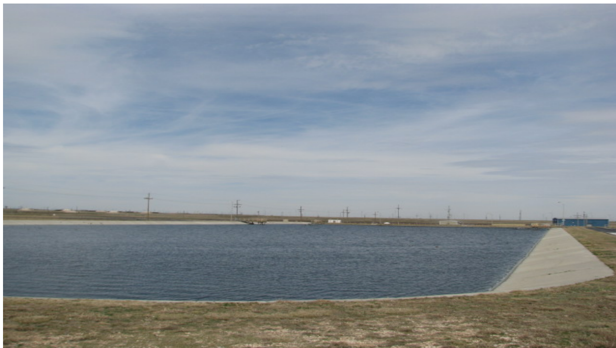
Figure 8.2 – Wastewater Treatment Facility, Facultative Lagoon
