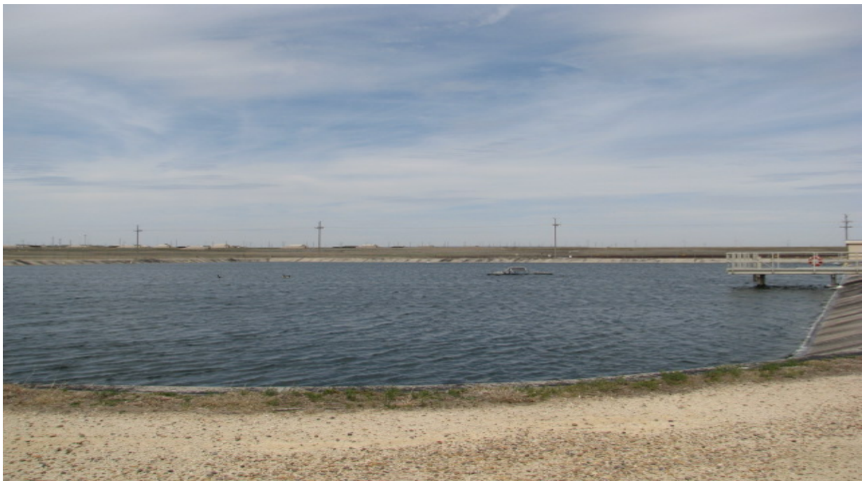
Figure 8.4 – Wastewater Storage Lagoon
