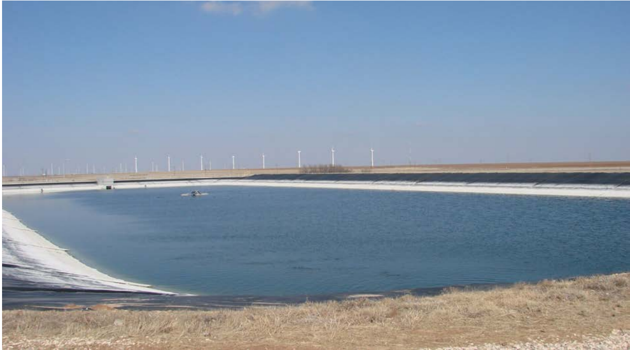
Figure 8.3 – East Wastewater Storage Lagoon
