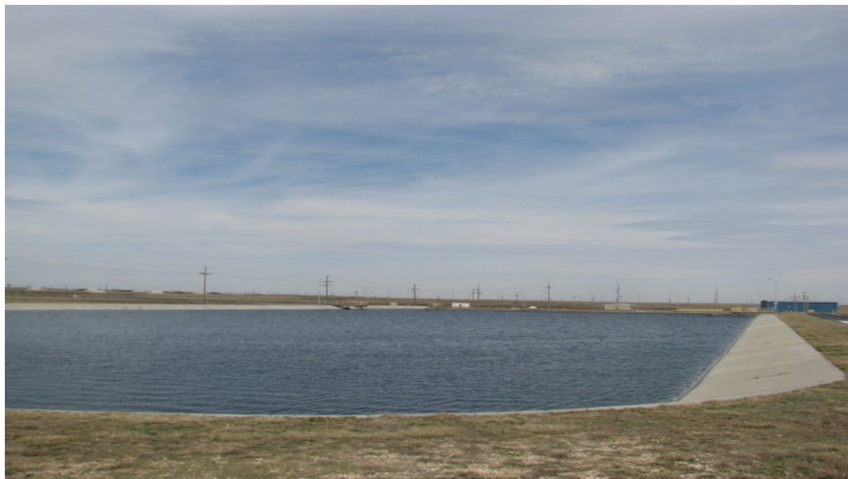
Figure 8.2 – Wastewater Treatment Facility, Facultative Lagoon
