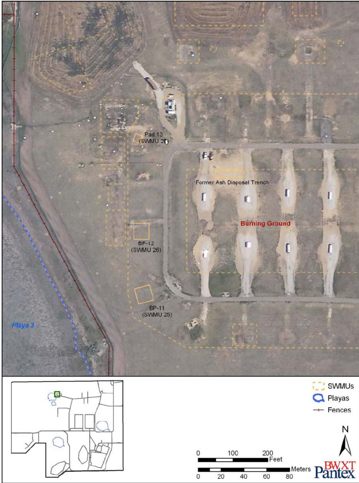
Figure 2-18. Burning Ground Former Ash Disposal Trench and SWMUs 25, 26, & 27
