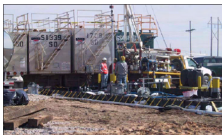
Injection of soybean oil into perched groundwater to enhance bioremediation
