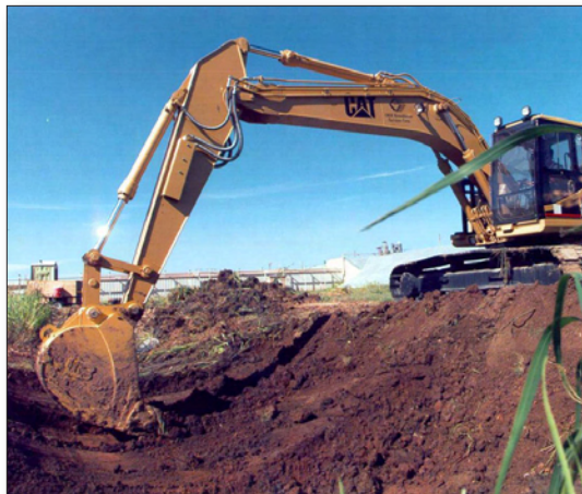
Excavation of ditch soils in Zone 11
