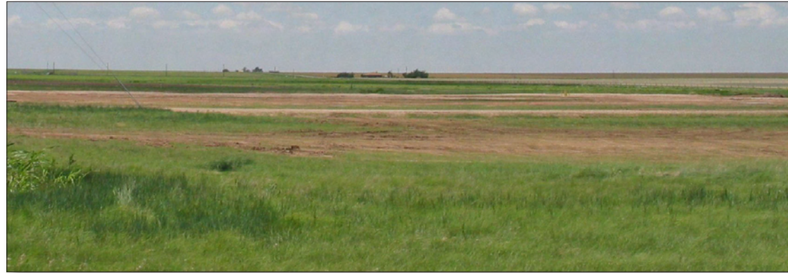
Old Sewage Treatment Plant (OSTP) after deactivation and decommissioning
