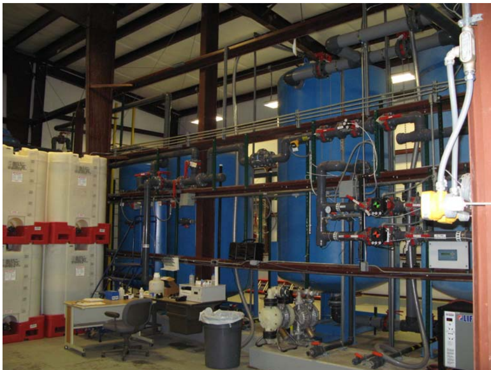
SEPTS Chromium and Boron Ion Exchange Units
