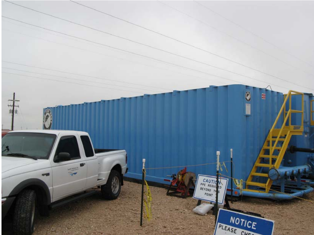
Makeup Water Storage Tanks
