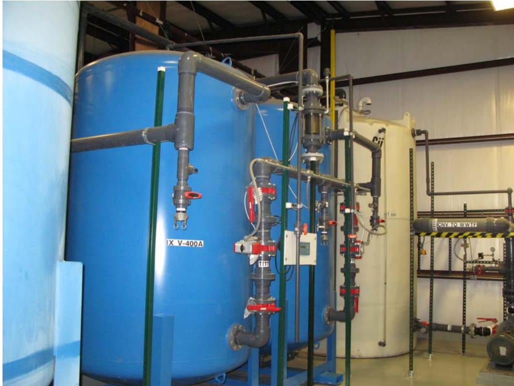
SEPTS Chromium IX Polishing Unit
