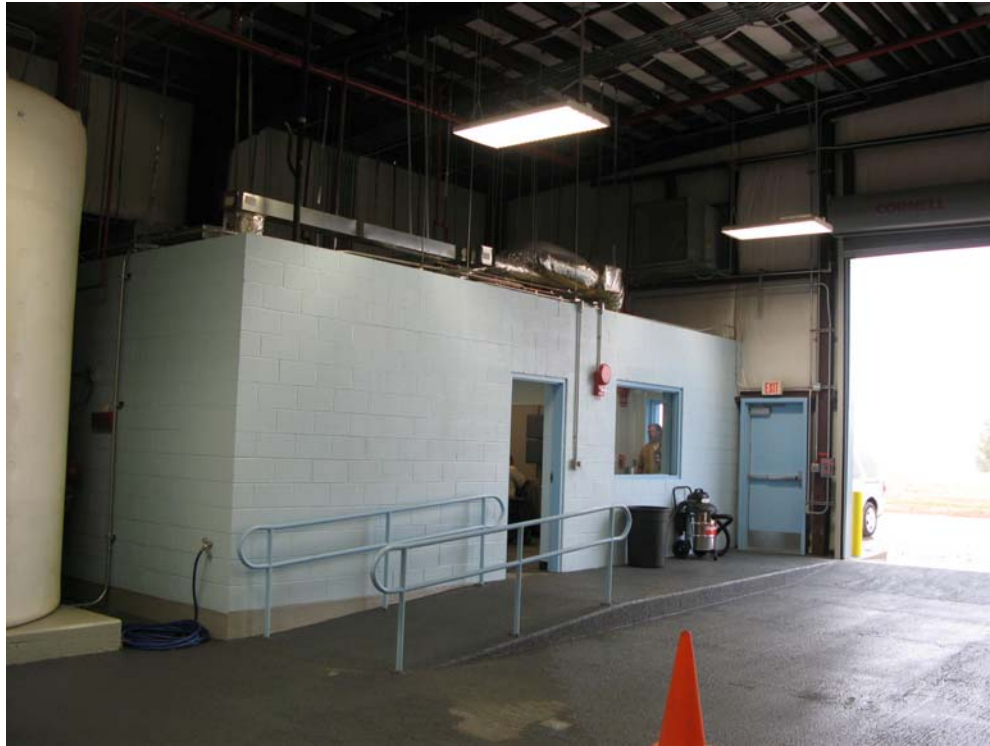
Exterior of Control Room (from within the Treatment Bay)
