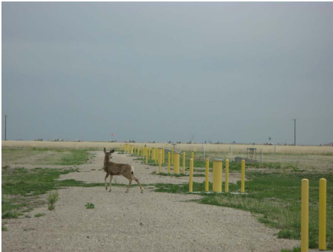
SEISB Injection Wells and Distribution Vaults
