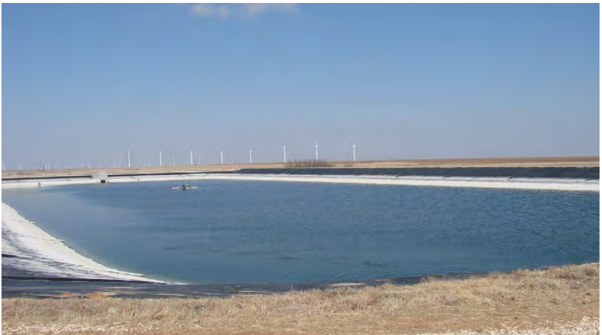
FIGURE 8.3 — East Wastewater Storage Lagoon
