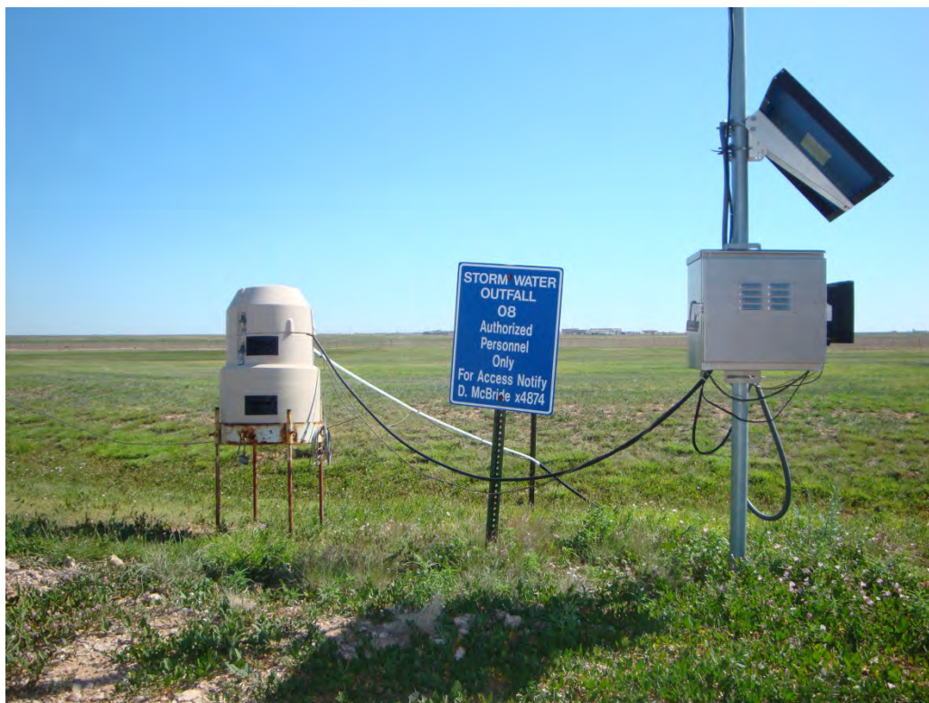
FIGURE 9.6 — Storm Water Outfall 08
