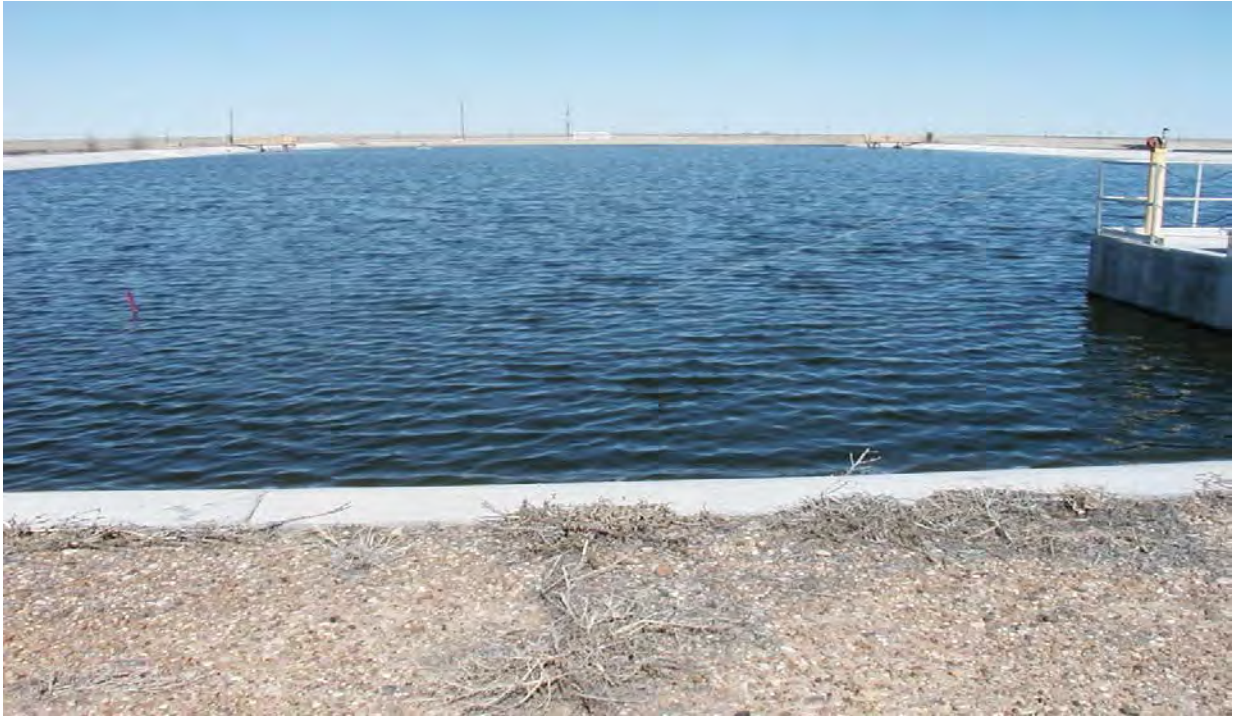
FIGURE 8.2 — Wastewater Treatment Facility, Facultative Lagoon
