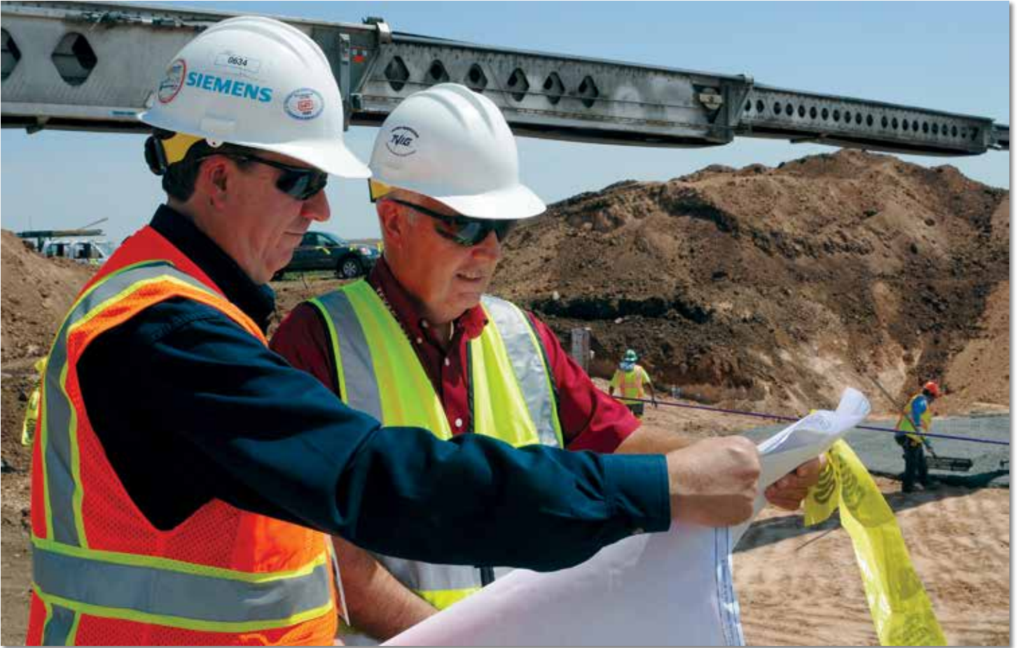
Chuck Mitchell, Siemens project manager, and Robert Cole, B&W Pantex Line Items program manager, review plans at the wind farm construction site. Photo by Larry Dov' Batchlear
