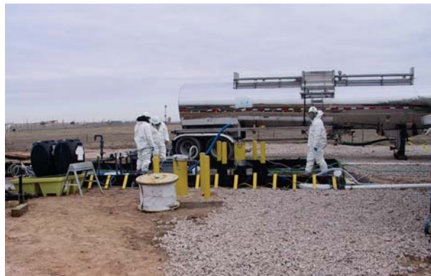
Injecting amendment into perched groundwater to create a permeable treatment zone.
