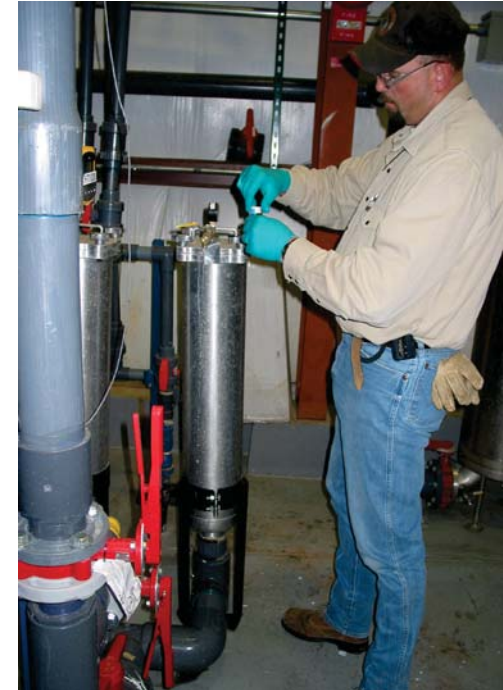
Sampling treated water from the pump and treat system.
