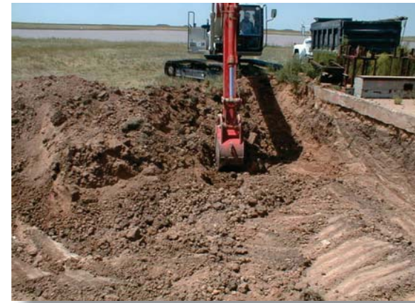
Excavation of soil at the Burning Ground.
