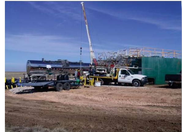
Preparing for injection of amendment to create a permeable treatment zone in perched groundwater.
