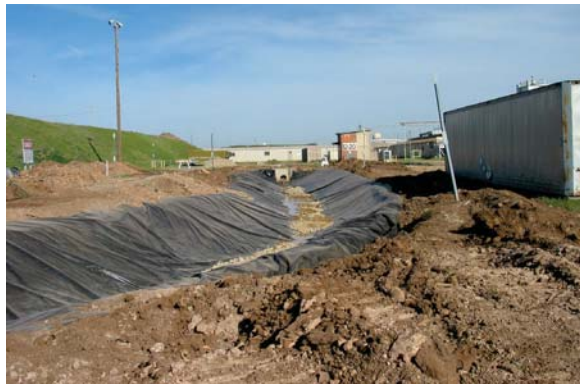
SWMU 5-05 after installation of the ditch liner.
