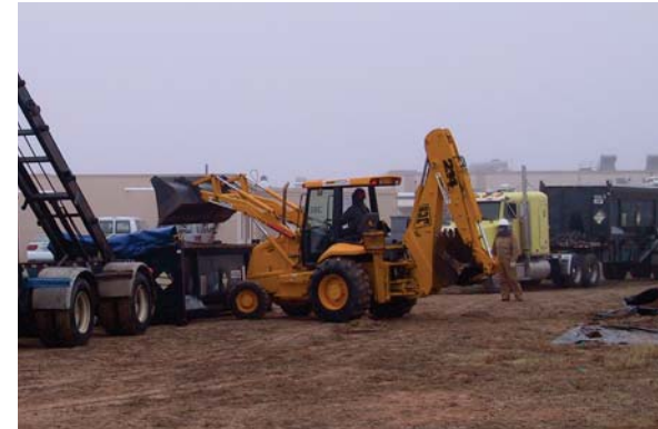
Loading of excavated soil into a roll-off container for disposal.
