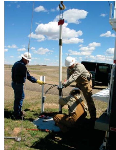
Sampling technicians making repairs to a well.
