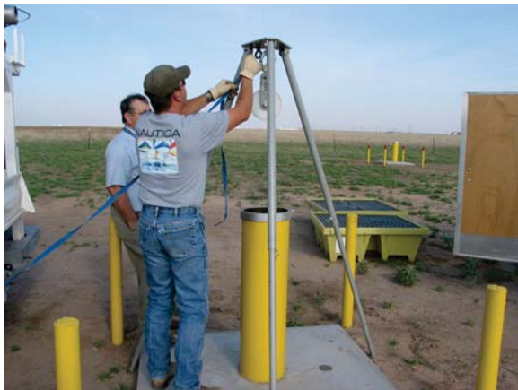
Sampling technicians preparing to video survey a well as part of the well maintenance program.
