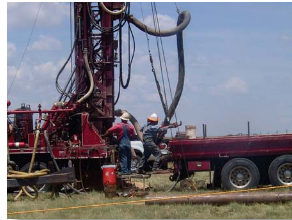
Drilling a new extraction well near Playa 1, July 2007.
