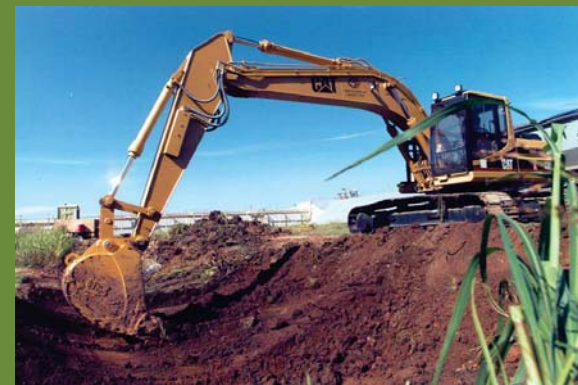
Excavation of ditch soils in Zone 11.
