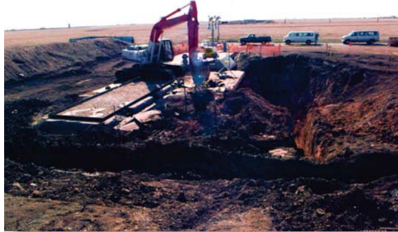
Excavation of soil at FS-5 during the interim corrective measure, 1997.
