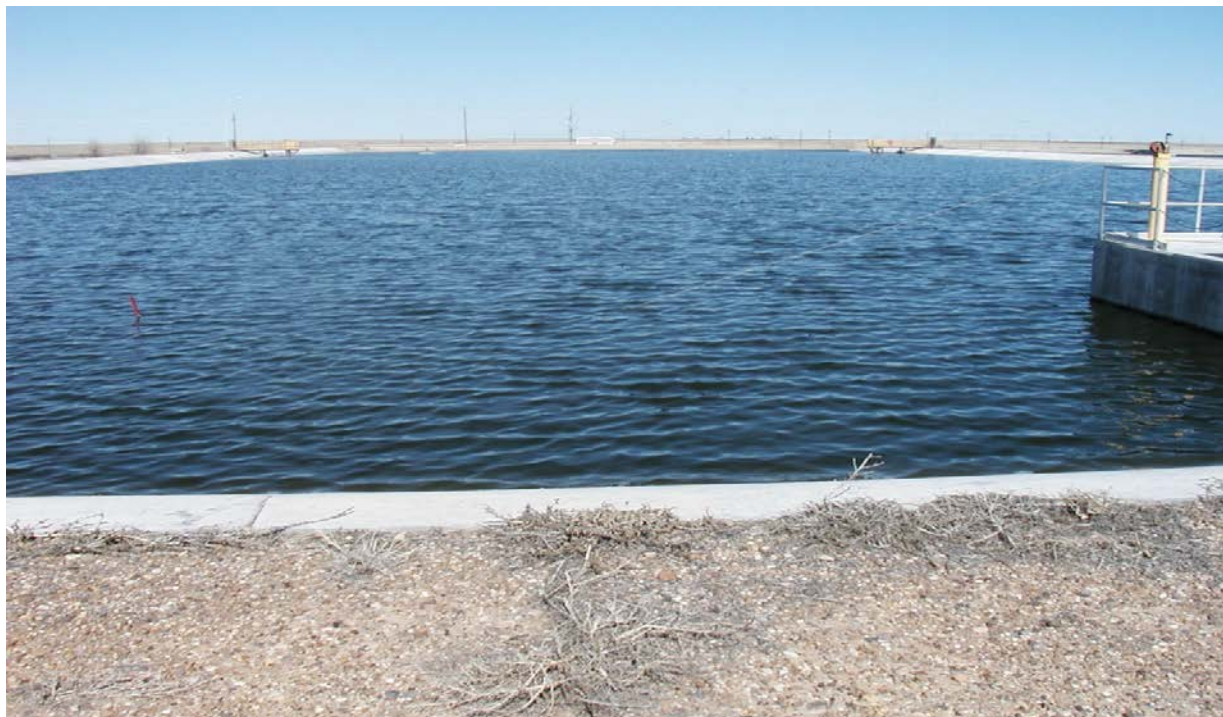
Figure 8.2 – Wastewater Treatment Facility, Facultative Lagoon
