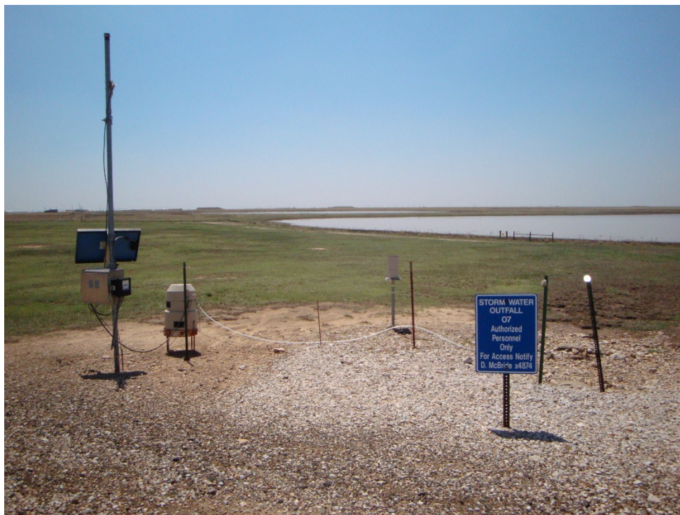
Figure 9.6 – Storm Water Outfall 07; Playa 3 in the Background
