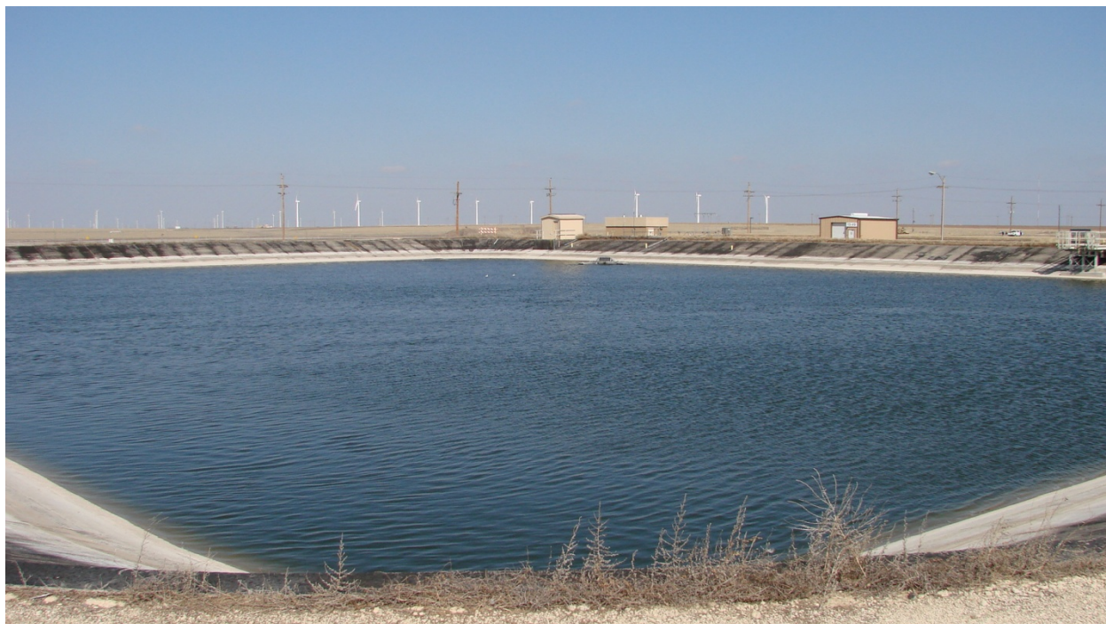
Figure 8.4 – Wastewater Storage Lagoon
