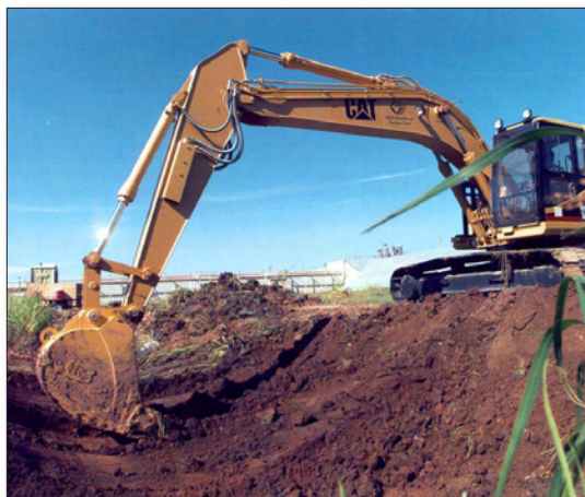
Excavation of ditch soils in Zone 11
