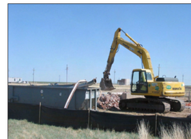
OSTP before remediation
